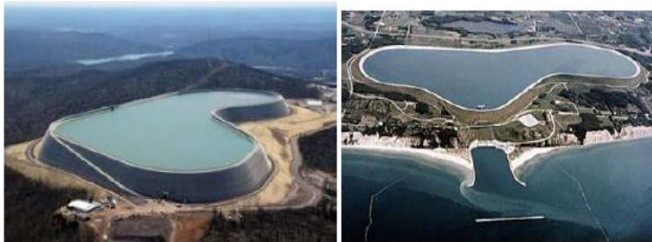
Concept and example of pumped-storage method of generating hydroelectricity
